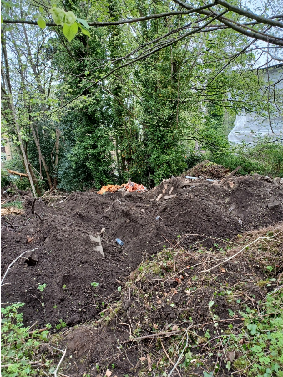
Image 3. Level changes in the rooting area of protected trees, caused by heaping of construction spoil within the woodland.
